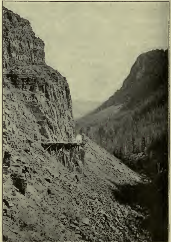
FIG. 12. — A rock cliff showing the cracks that extend through the rock; also, at the base of the cliff, a large pile of rock fragments that have been loosened by frost, and have fallen down the steep slope.
